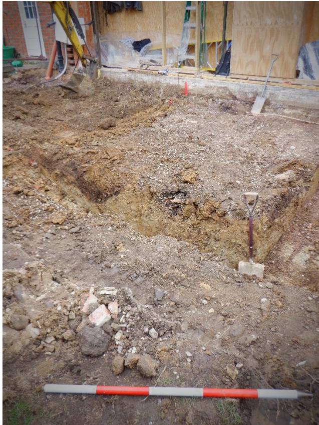
Plate 4. Foundation trenches (looking North)
