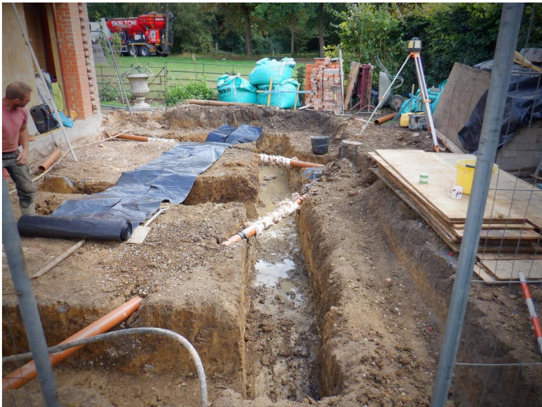
Plate 6. Foundation trenches (looking East)
